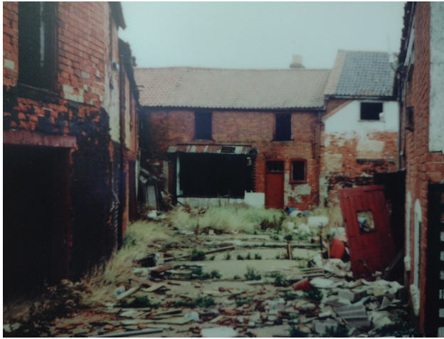
Figure 1. Tower curing works derelict, Great Yarmouth (1990s) @ Norfolk Museum Service.
